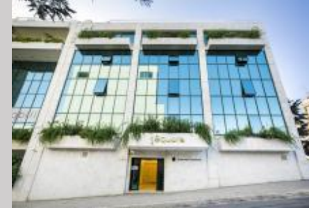
27, Alexandrou Pantou Street, Kallithea, office building, 1.358,97 m 2
