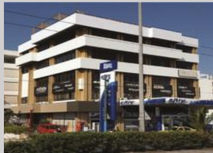
42 Poseidonos Avenue, Kallithea, mixed use building, 1.907,47 m 2
