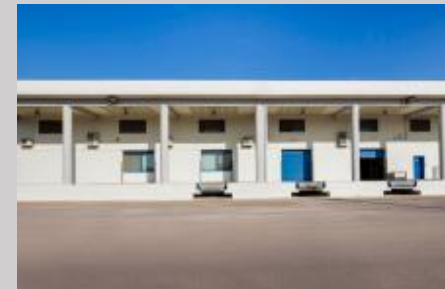
65, Loutrou Street, Acharnes, logistics building, 3.974,75 m 2
