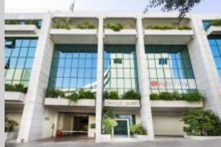
25, Alexandrou Pantou Street, Kallithea, office building, 6.637,42 m 2
