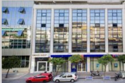
2A, Argyroupoleos Street, Kallithea, office building, 3.915,33 m 2
