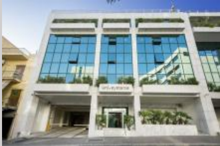
19-23, Alexandrou Pantou Street, Kallithea, office building, 6.806,03 m 2
